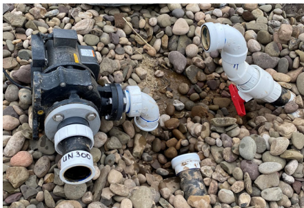
5. Turn pump over and drain water out of pump body
